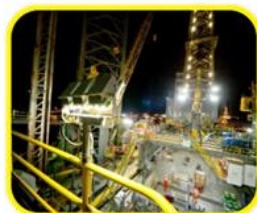
Petrol Process Factory
