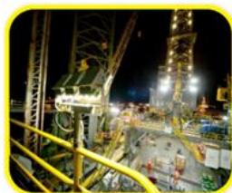
Petrol Process Factory
